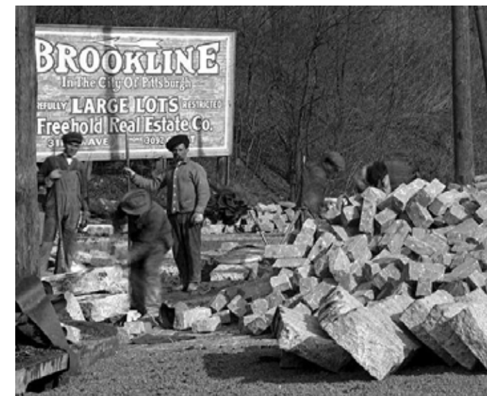
Street paving in the early 1900s was often done using Belgian Blocks. This shows construction workers cutting stone blocks at the corner of West Liberty Avenue and Cape May in 1915.
